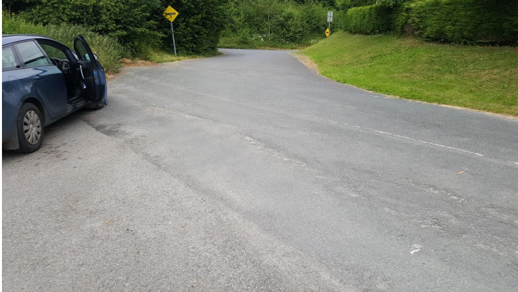
Plate 12.7 Access junction on local road – looking north along local road
